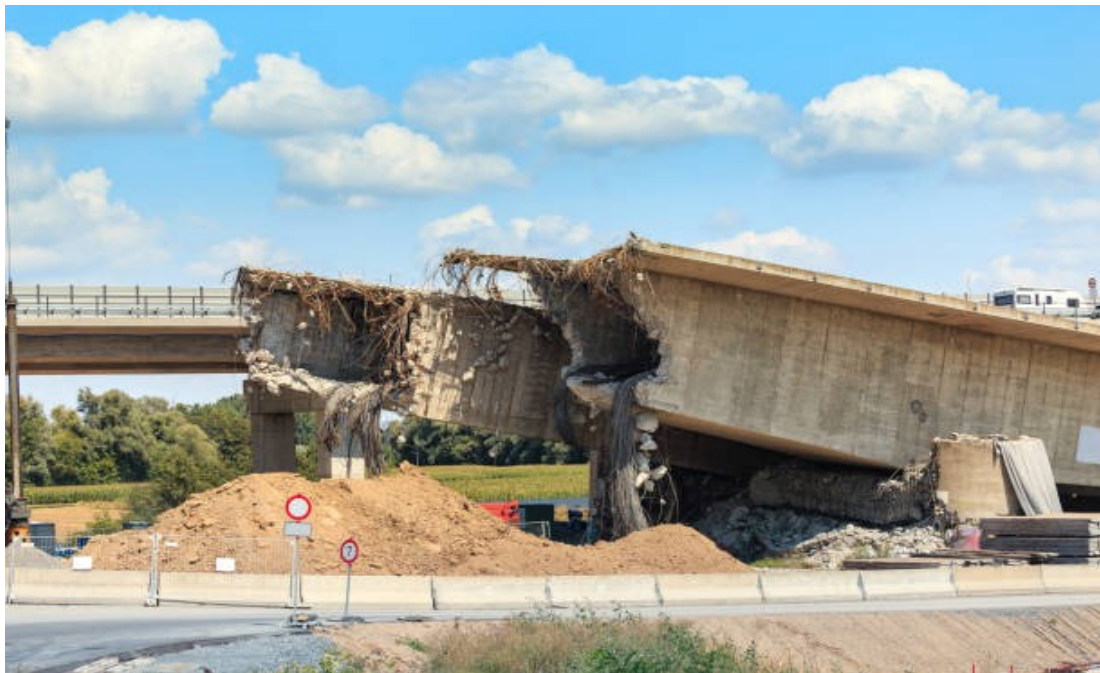
Image Credit 03: istockphoto frantic00 (Destroyed road bridge)
