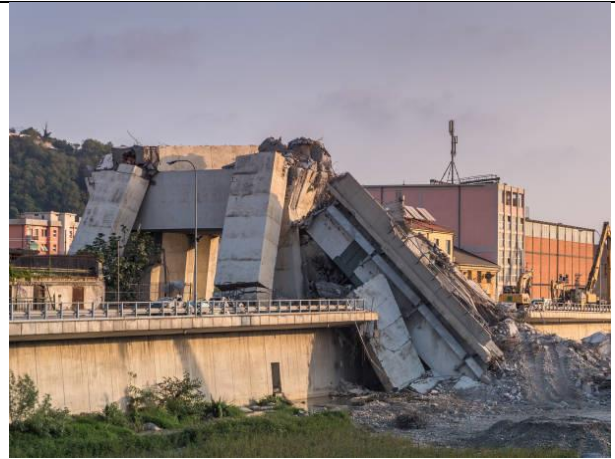
Bridge Collapse due to Cyclones
